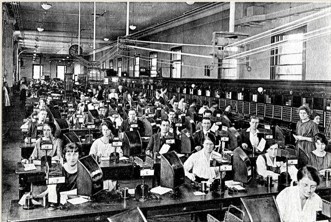
FOURTH FLOOR. Intercommunication Switch for Metropolitan Offices.
