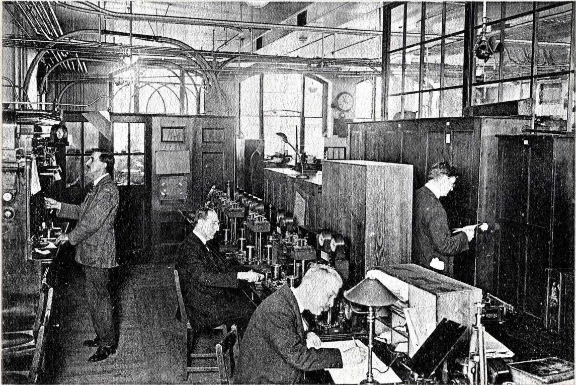
INTERNATIONAL CABLES. REPEATER, AND TEST ROOM.
