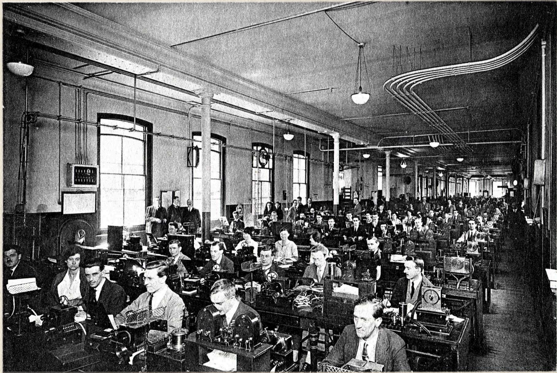
MAIN GALLERY OF CABLE ROOM. (International, Cable and Wireless.)
