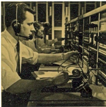
Trunk test desk: throughout the day and night technicians man testing positions from which a fault on any circuit can be rapidly identified and located.
