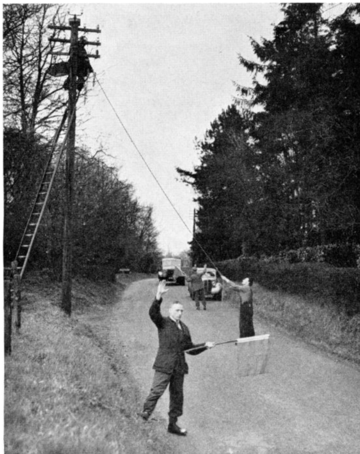
FIG. 12. —EMPLOY FLAGMAN AS AN ADDITIONAL PRECAUTION WHEN WORKING ACROSS BUSY ROADS. TWO FLAGMEN MAY BE NEEDED AT ROAD BENDS OR JUNCTIONS.
