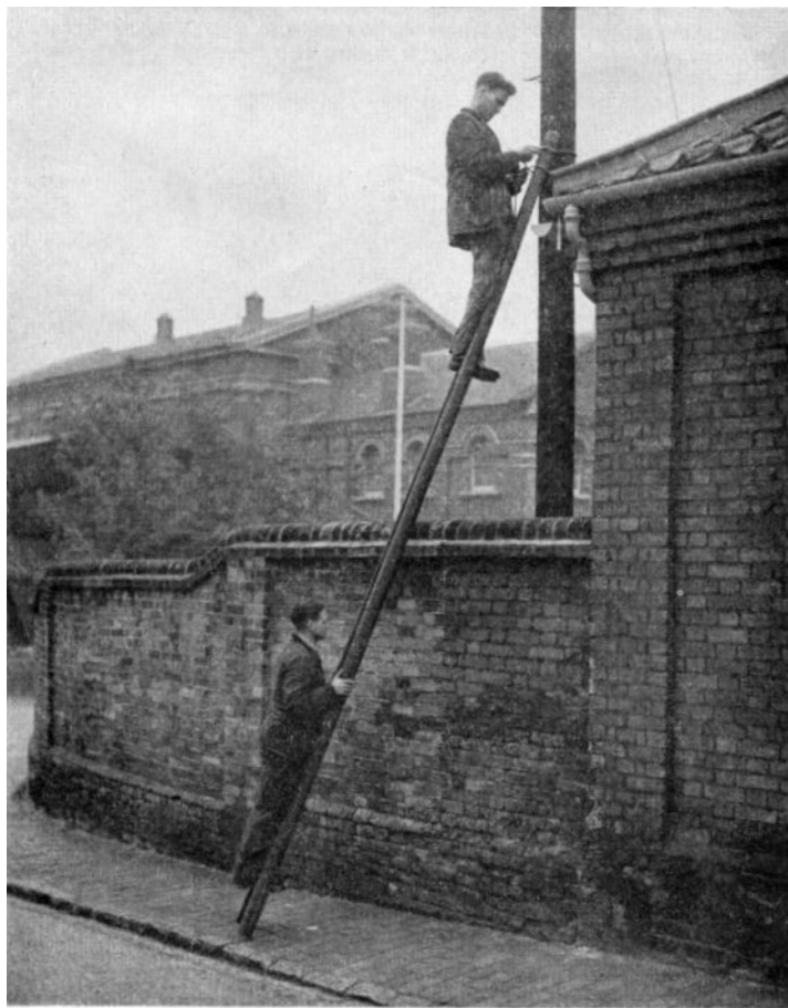
FIG. 7.—If good foothold is not obtainable, and in busy streets, have man at foot until ladder is securely fastened at top.
