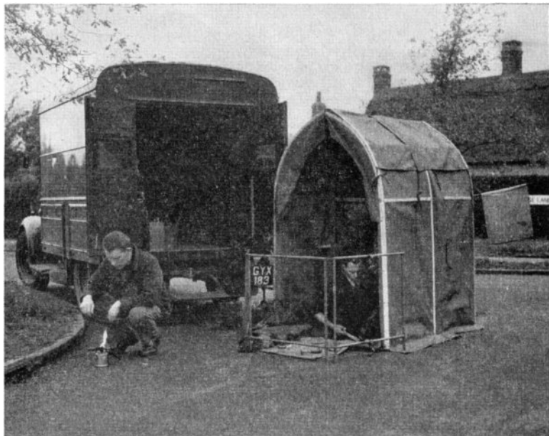
FIG. 17.—NEVER LIGHT A BLOWLAMP IN A MANHOLE, FOOTWAY BOX, VEHICLE OR NEAR INFLAMMABLE MATERIAL
