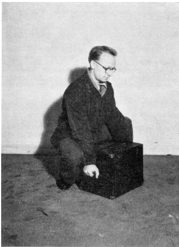
FIG. 19.—AT COMMENCEMENT OF LIFT THE BACK SHOULD BE STRAIGHT AND ARMS FULLY EXTENDED
