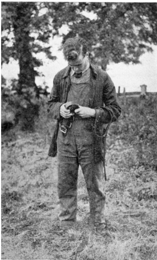
FIG. 11.—EXAMINE SAFETY BELT BEFORE USE. REJECT IF LEATHER BADLY CRACKED OR STITCHES BROKEN.
