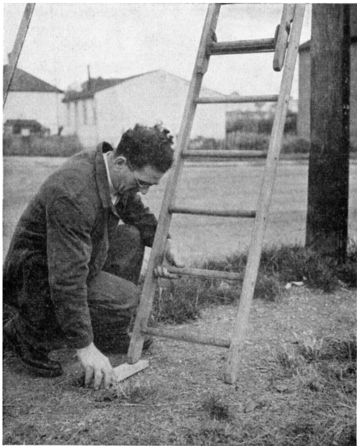
FIG. 6.—GET FIRM FOOTHOLD FOR LADDER AND ERECT AT MODERATELY STEEP ANGLE. (4 : 1)
