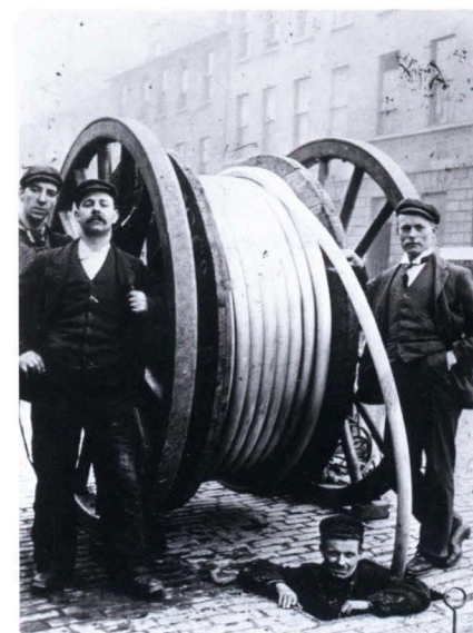
Above: An underground cable-laying gang c.1910. Prior to the advent of underground cabling, the urban skyline was an unsightly tangle of derricks and open wires. Moving the infrastructure underground improved both the reliability of the network, and the visual environment.
