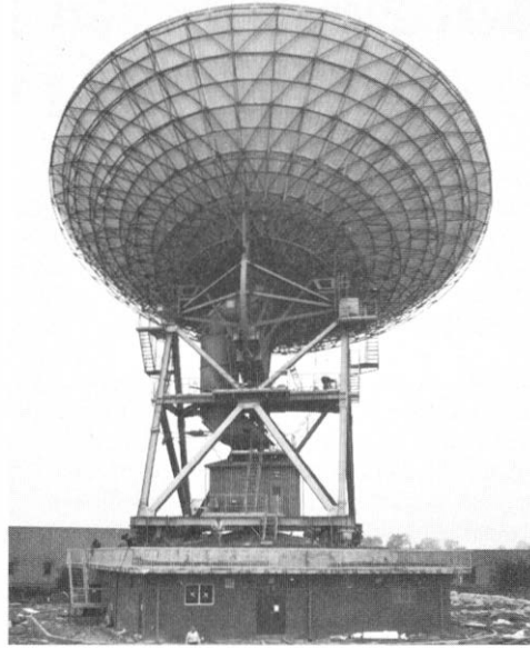
Madley's first Aerial System with a view of the beam waveguide and the relatively lightweight backing and support structure.
