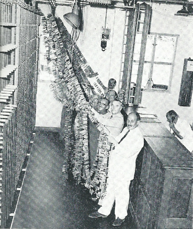
The pegs are withdrawn, the lines are connected, and the new exchange at Dar-es-Salaam is in service
