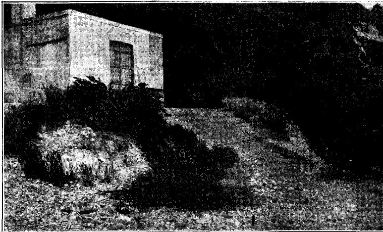
(6) ST. MARGARET'S SUBMARINE TELEGRAPH AND TELEPHONE CABLE HUT, NEAR DOVER.
