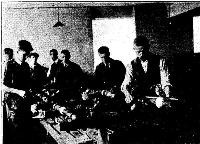
8.—JOINTING SCHOOL—WIPING JOINTS.
