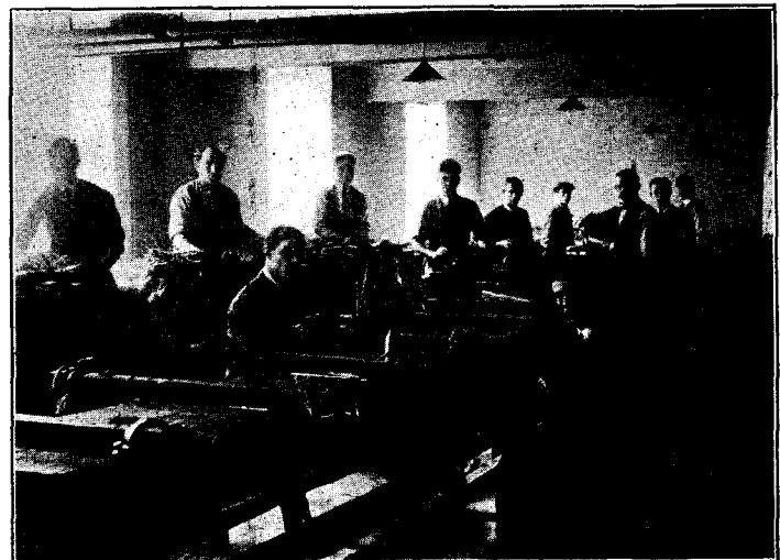
7.—JOINTING SCHOOL—MAKING CONDUCTOR JOINTS.
