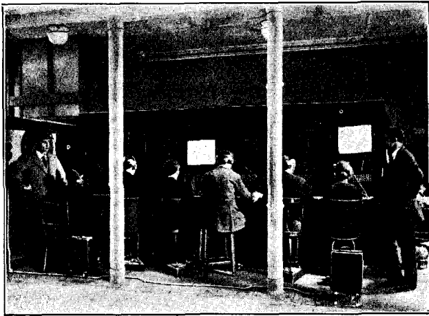
FIG. 1.—THE OLD MANUAL SWITCHBOARD INSTALLED 1907, DISMANTLED JUNE, 1925.
