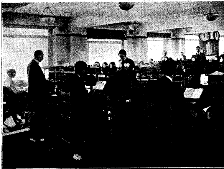
WHEATSTONE TABLES. TRAFFIC OPERATING ROOM (FOURTH FLOOR).
