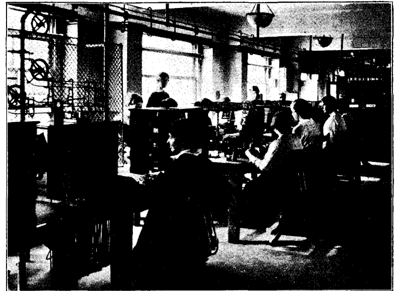
BRANCH WIRES, CONCENTRATION BOARD AND CIRCUITS.
