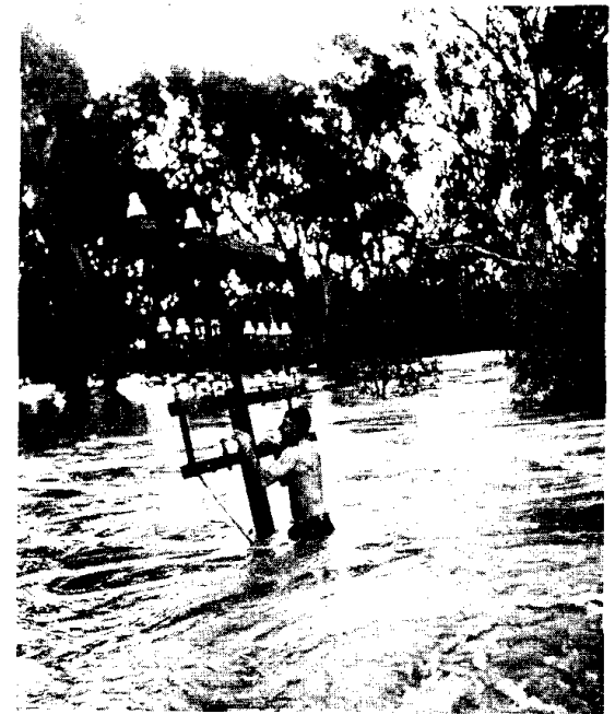
Flood repair work in Maitland, N.S.W.
