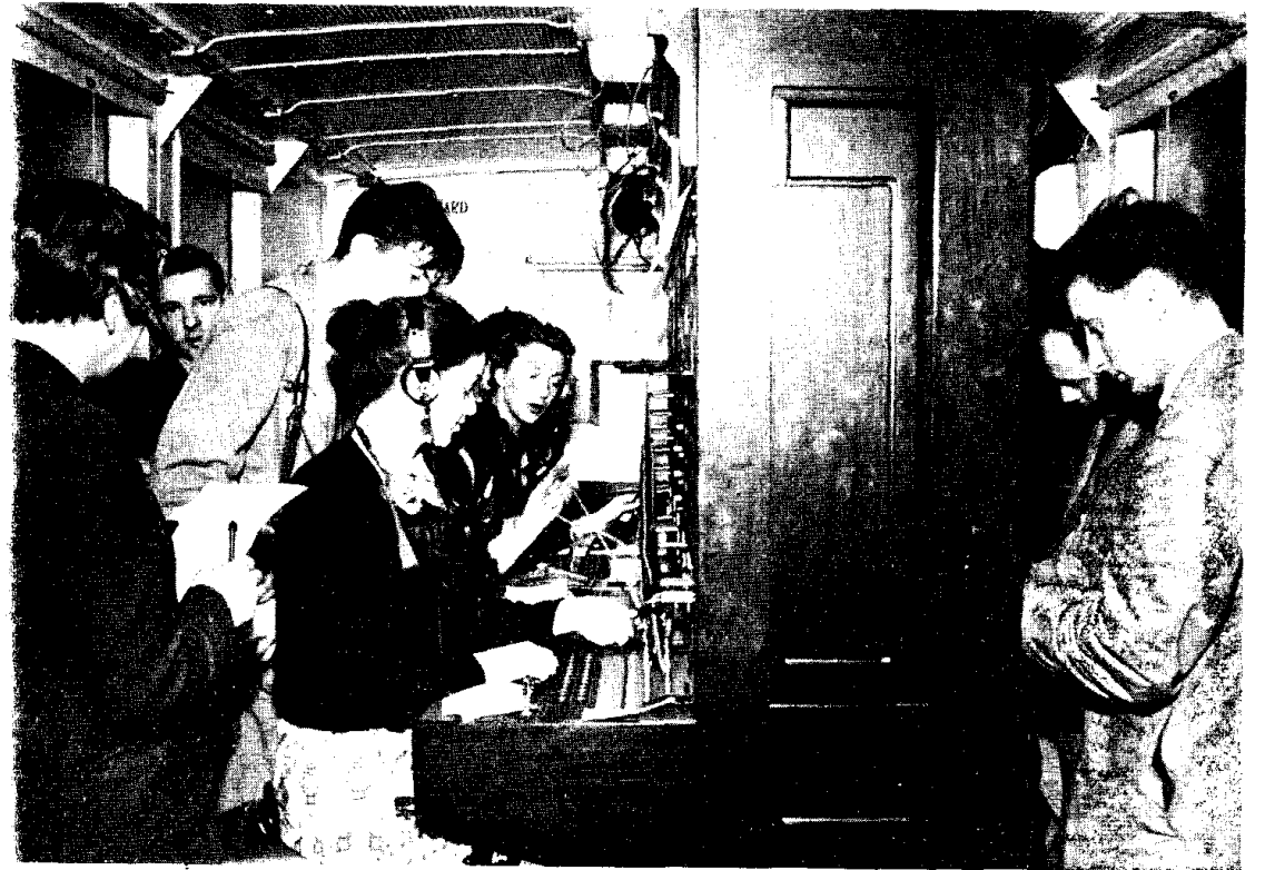
Three-position switchboard in the caravan Courtesy of Ovens & Sons, Wishaw
