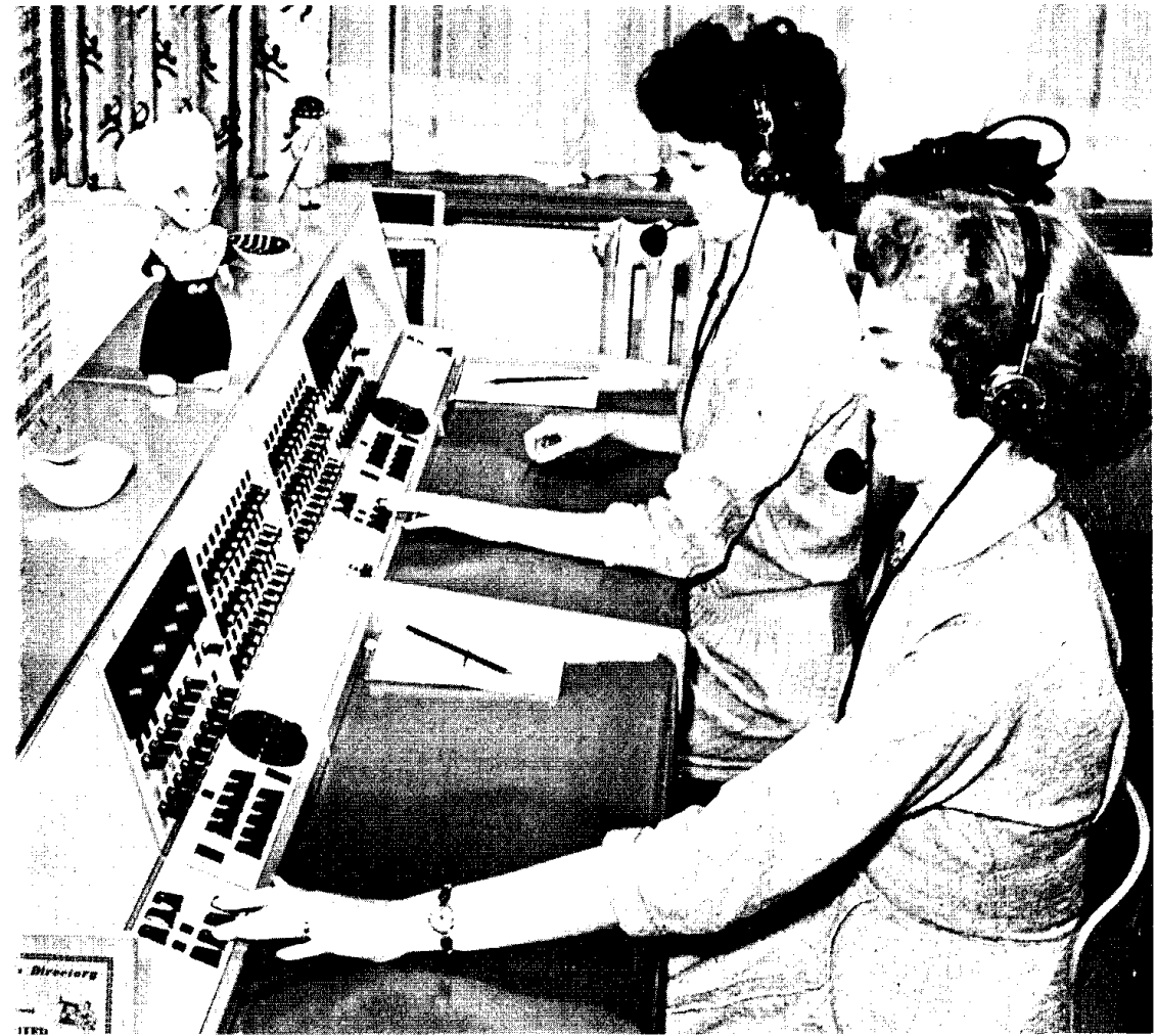
Fig. 4: Cordless switchboard, Hull Guildhall (Courtesy of Hull Daily Mail)
