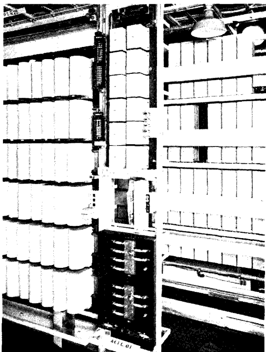
Fig. 7: Rack of power plant installed in line with telephone switching equipment
