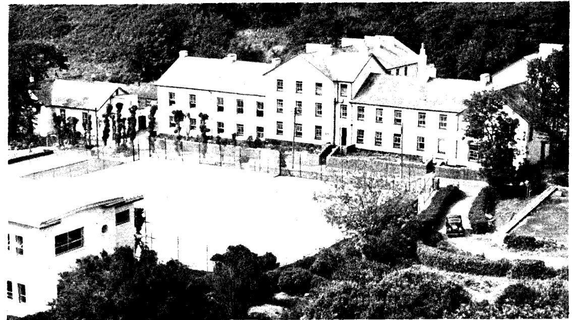
Cable & Wireless Engineering School at Porthcurno: single staff quarters and new instructional block in left foreground
