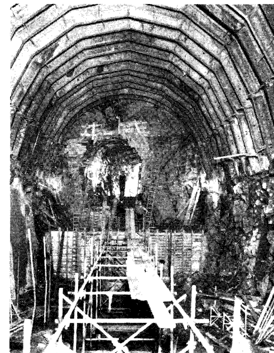
Fig. 2 : The tunnel under construction—"The Cathedral"
