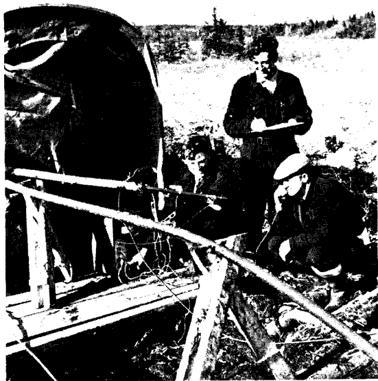
Some of the Post Office team splicing the land cable in Newfoundland
