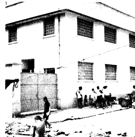
The new Quarry Bay exchange
