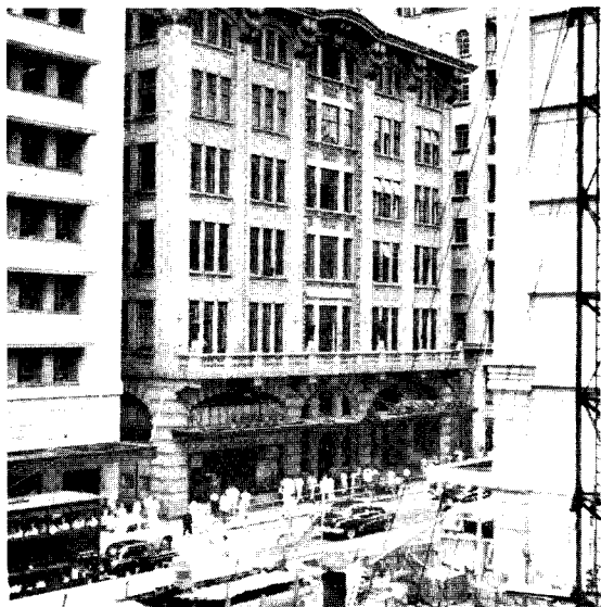
Head Office of the Hong Kong Telephone Company and Central exchange
