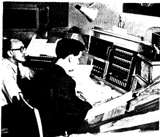
The Terminal Manager's Control Room: on the desk are mounted the keyboards controlling the "Teletalk" system and passenger movement through the South East Face Building
