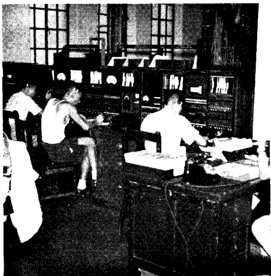
Part of the test desk Victoria exchange
