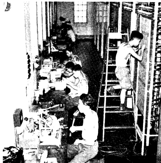
Adjustment bench at Central exchange
