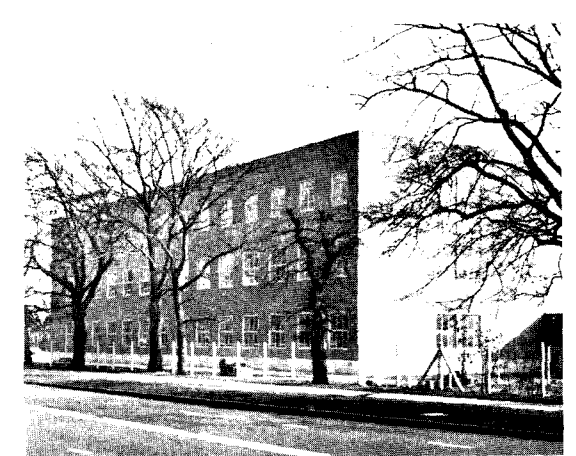
Skyport Telephone Exchange
