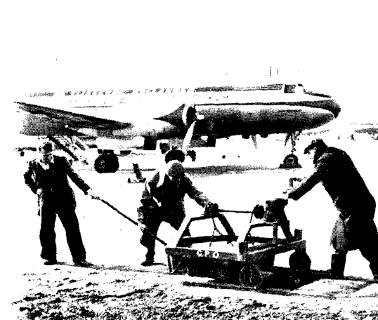
Manhole cover mechanical lifter
