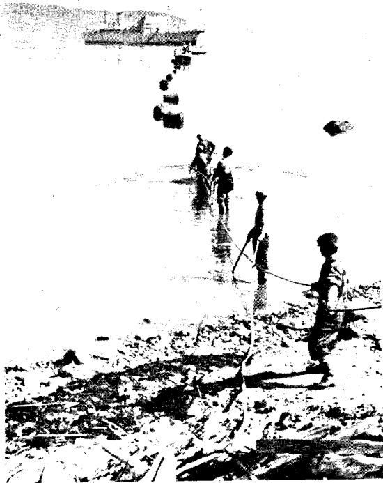
H.M.T.S. Monarch , which is laying all the cable, lying at anchor off Clarenville, Newfoundland, while motor launches pull the first shore ends from her holds. Monarch , built for the Post Office in 1945, is the only cable ship afloat capable of carrying the 1,500 nautical miles of cable, which must be laid in one piece across the deepest part of the Atlantic
