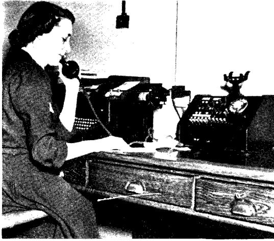
A small P.B.X. serving a Government department; operating combined with typing duties
