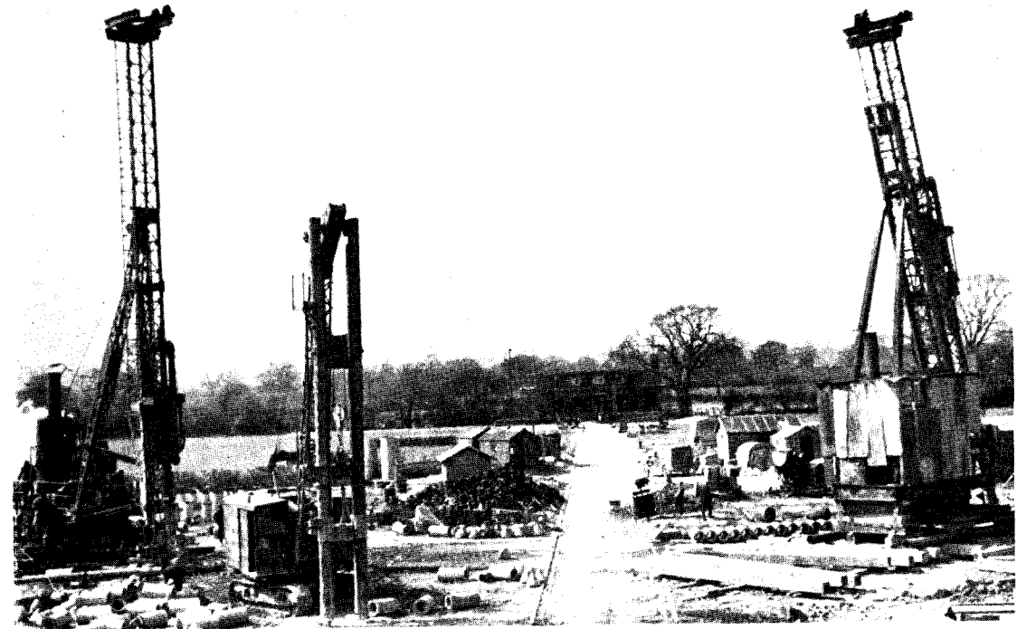
Fig. 2 : Piles being driven : for each foundation a cluster of piles was capped by a massive concrete block
