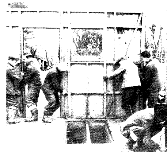
Fig. c : Front end section (old type) B building being lifted into position
