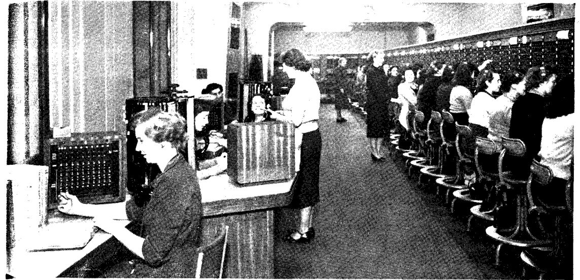
A large P.B.X. serving Government departments, showing four enquiry positions on the left
