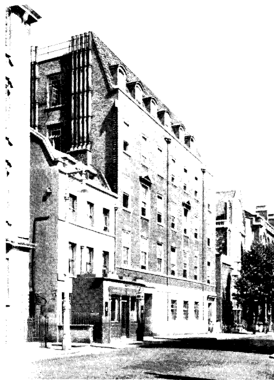
A modern telephone exchange: Mayfair Building, London, which contains four exchanges handling a total of some 300,000 calls a day
