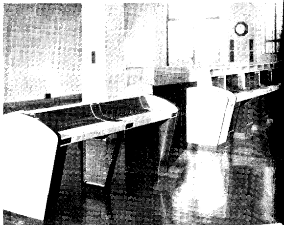
Two incoming positions and monitorial suite with pneumatic tube terminal
