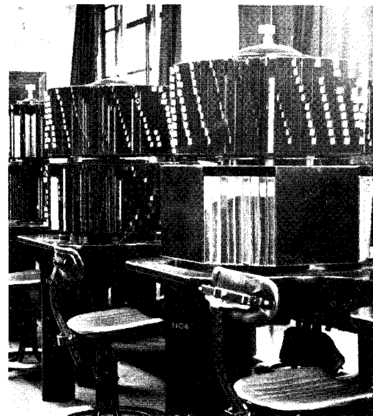
Trunk and toll exchange Birmingham: Directory Enquiry positions, showing amendments carried on drums instead of in loose-leaf books
