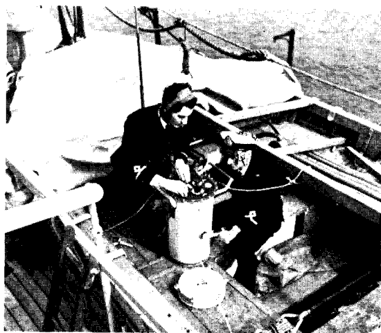
Portable radio transmitter and receiver being tested in a life-boat. Power is provided by a generator driven by turning the crank handles
