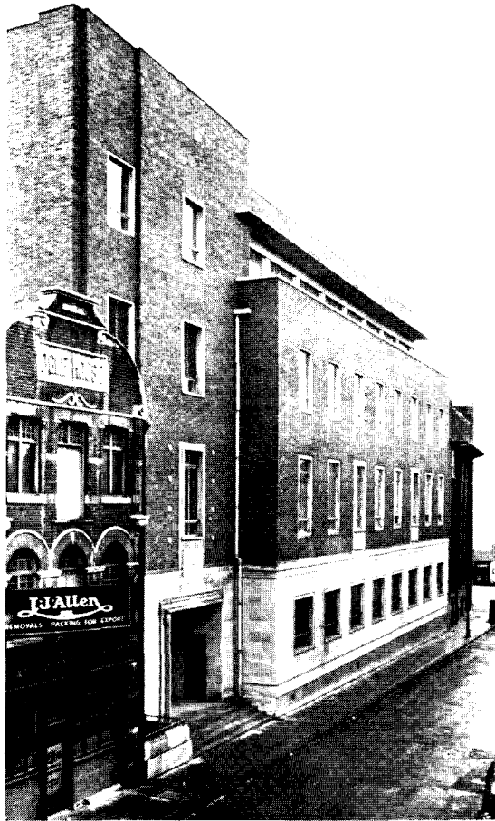
Southampton Telephone Exchange, Ogle Road (By courtesy of the Ministry of Works)
