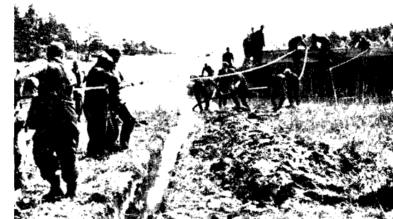
"Alert" landing the shore end of the Sweden-Gotland power cable at Vasterrat
