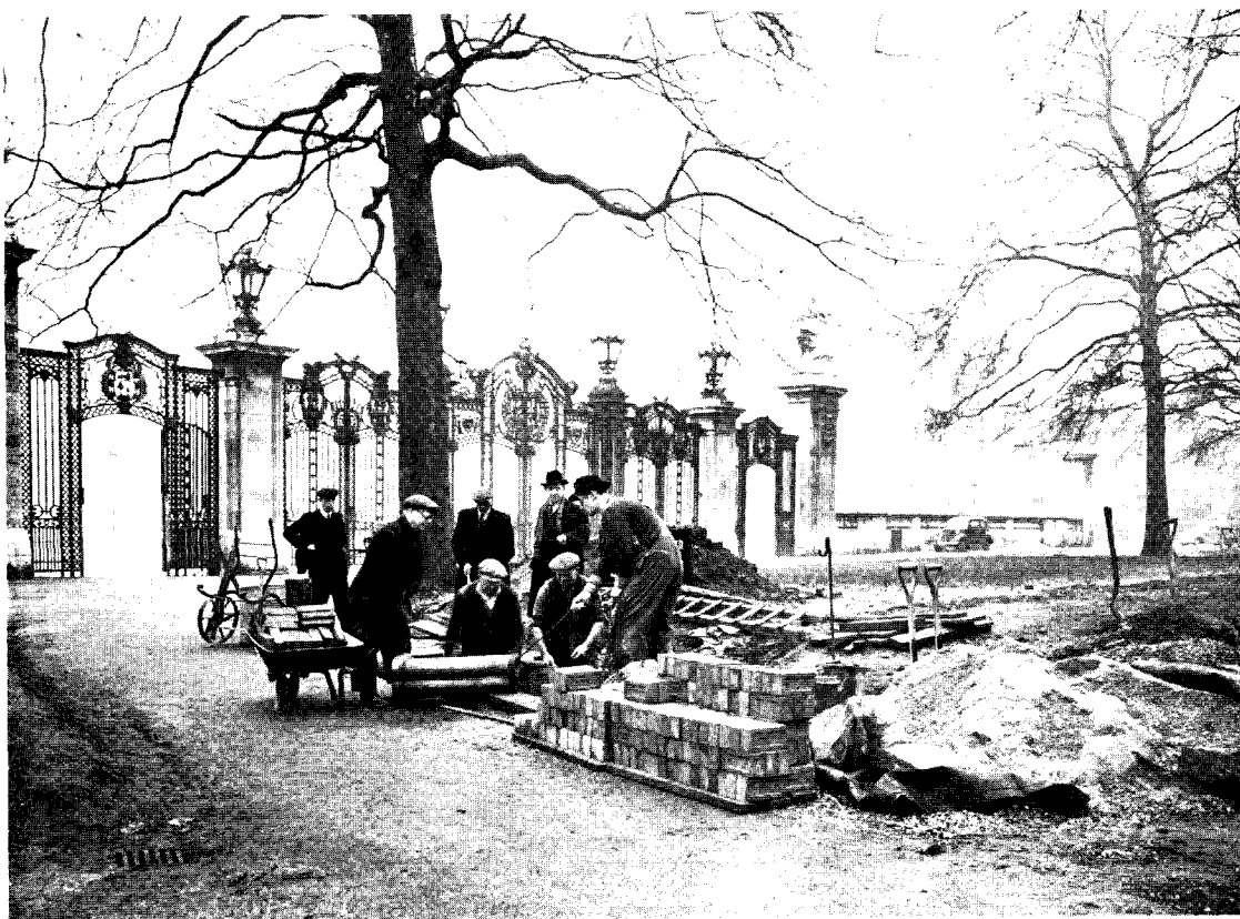
Completion of first duct work at Canada Gate, Green Park
