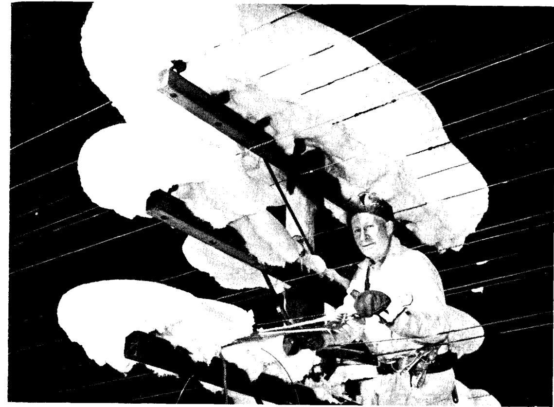
Linesman at work on communication pole (Photo, by courtesy C.P.R.)
