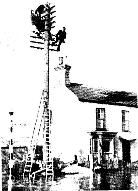
Providing emergency service at Sutton-on-Sea
