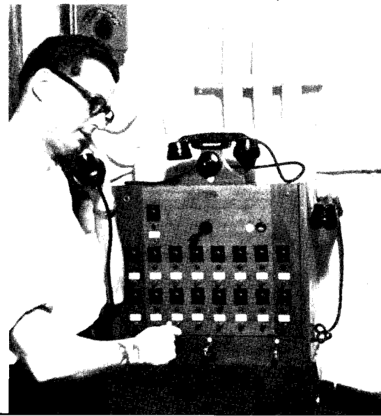
Switch panel in ship's main kitchen (By permission of the Cunard Steamship Co., Ltd.)
