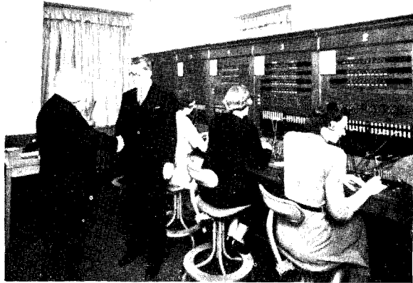
Mr. H. M. TURNER, Telephone Manager, formally hands over Coronation exchange to Mr. N. SIZER, M.B.E., Assistant Chief Engineer, Ministry of Works.
