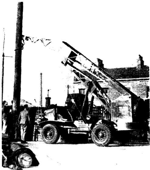
Initial stage in recovering a 50-foot stout pole Photo. F. K. Bottomley
