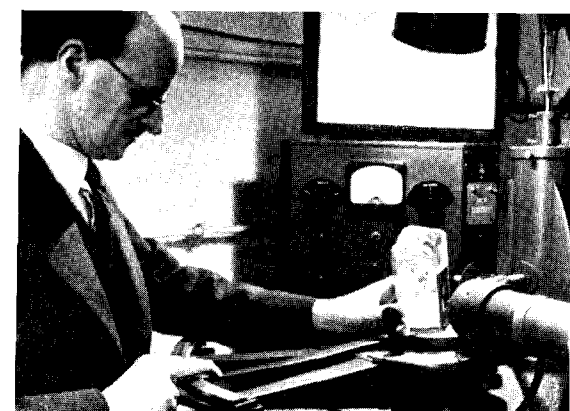
Testing orientation of cut surface of crystal with X-ray spectrometer
