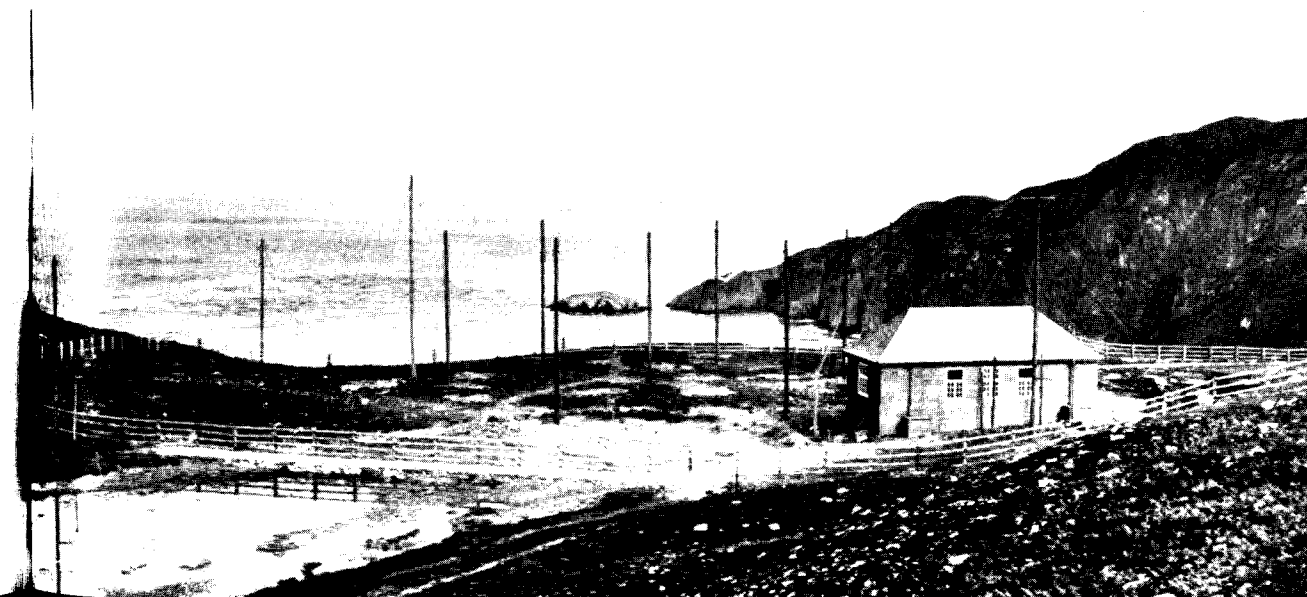
A typical multi-channel V.H.F. radio station
