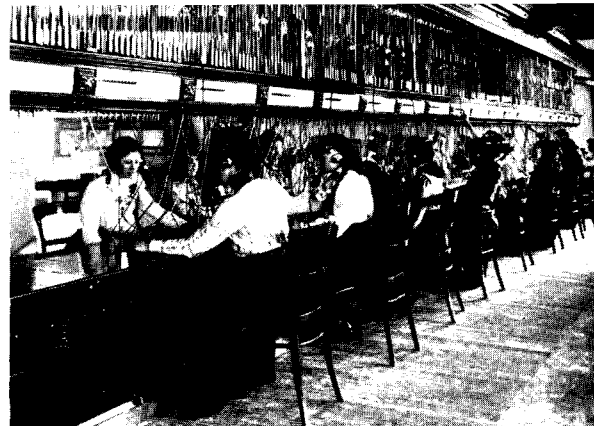
Glasgow Central, the first multiple switchboard, 1880
