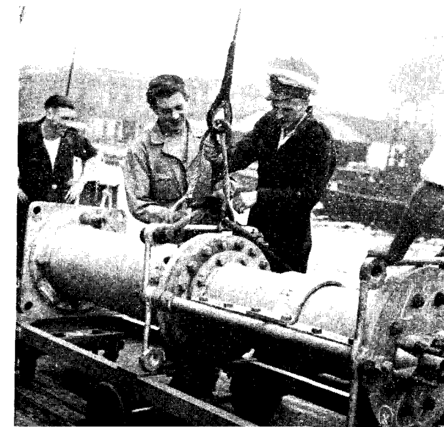
GENERAL VIEW OF A REPEATER
