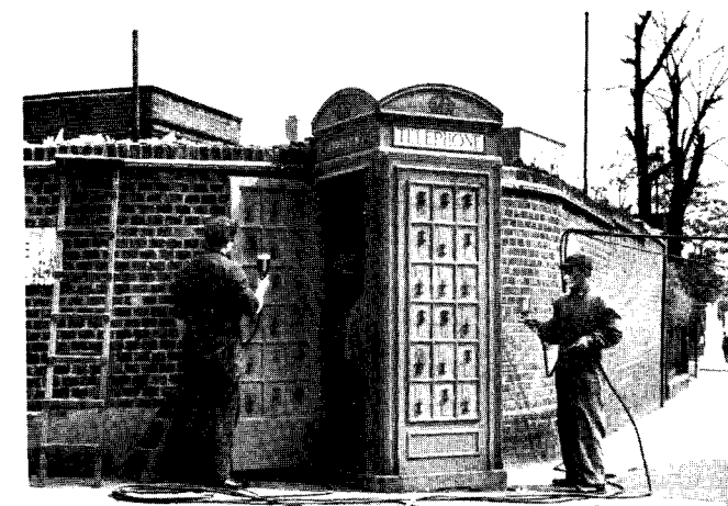
Fig. 5. Painting a kiosk with the spray-gun
