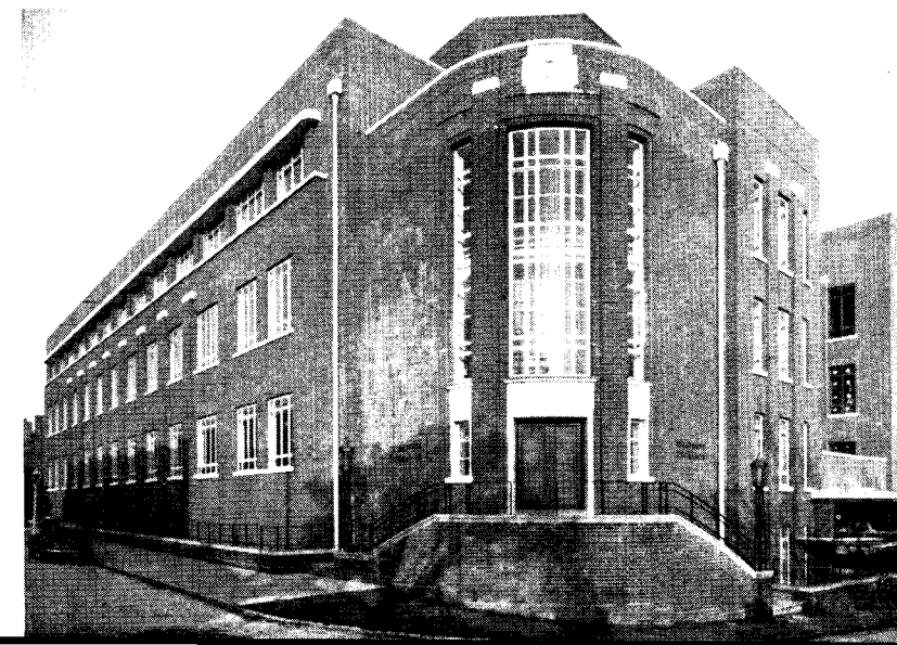
"Thanet" Telephone Exchange
