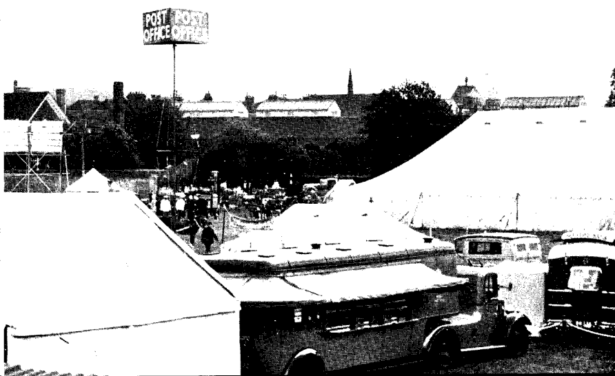
GPO 2 at the Royal Horse Show, Richmond. The extensible mast is anchored to the ground and the vehicle. Mast and sign pack into small space when not in use.
