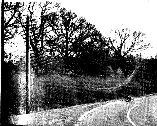
Some poles were broken at the top, others at the base.
