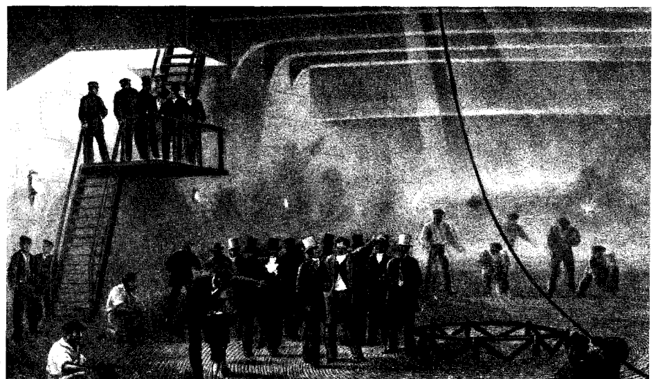
Laying the Atlantic cable in 1865. Coiling the cable into the after tank on board the Great Eastern at Sheerness. Visit of H.R.H. The Prince of Wales
