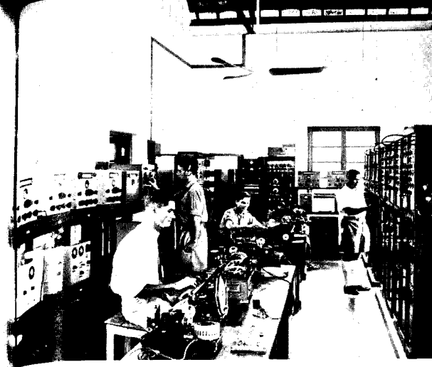
Cable & Wireless Station, Colombo (Interior: Porthode Receiving Station)
