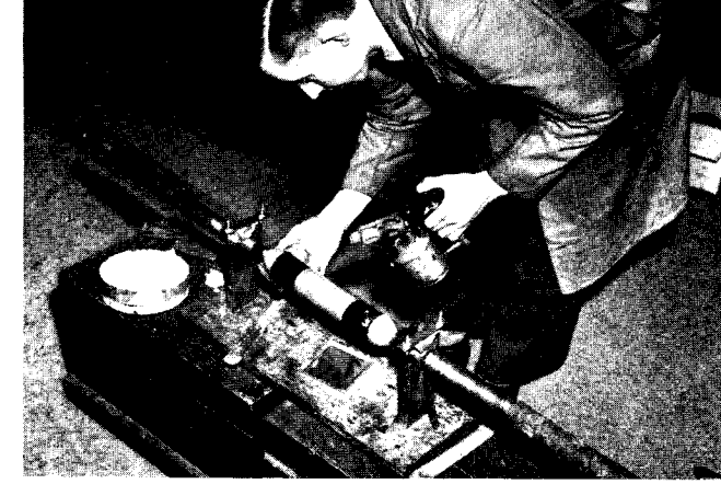
A student at the Cable & Wireless London Training School making a wiped joint in a lead-covered paper-core cable
