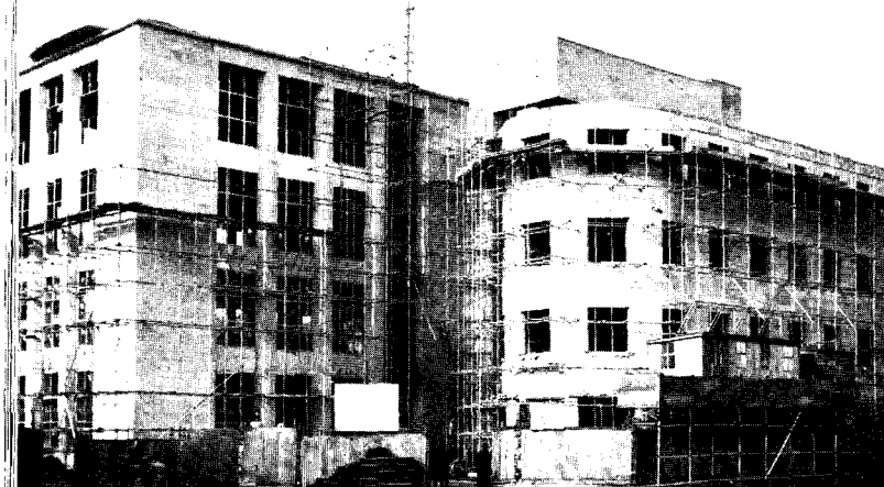
Fig. 2. Fountainbridge Telephone Exchange under construction (By courtesy of the Ministry of Works)
