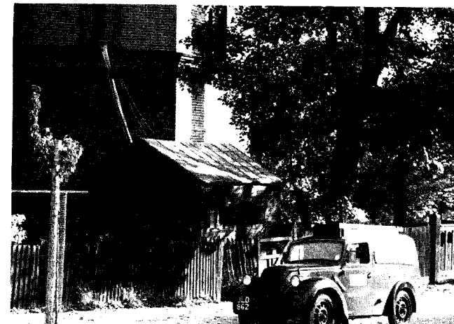
Below: The radio hut at the foot of the water tower at Shooters Hill
