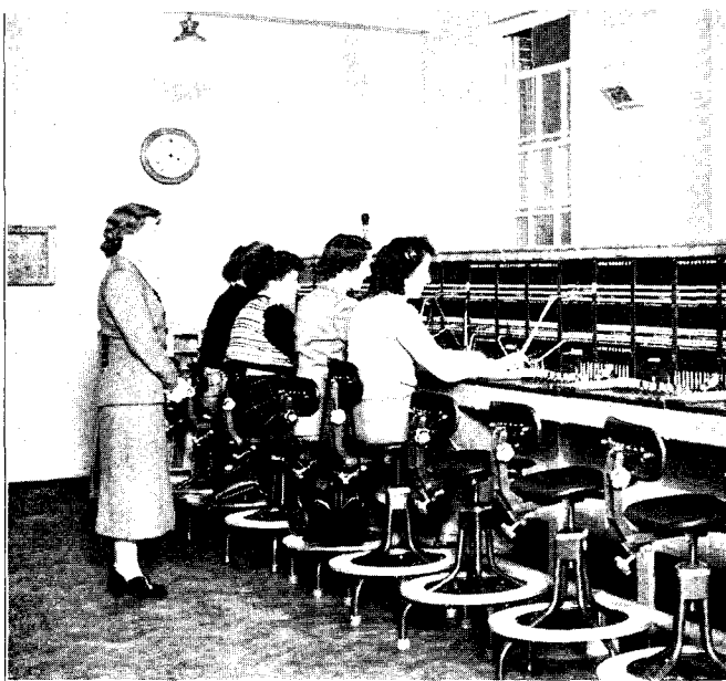
Part of the new switchroom at Gainsborough
