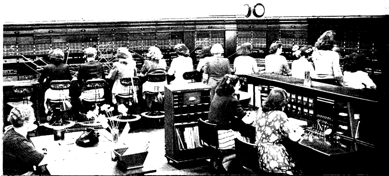
The new switchroom
