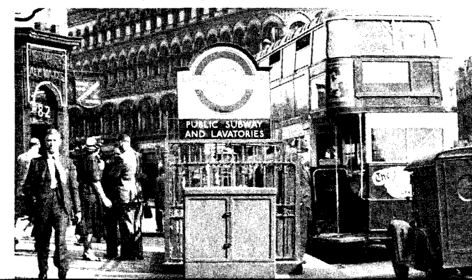
Fig. 2. Flexibility cabinet installed near the subway at Mansion House Station, London, and sited not to cause obstruction
