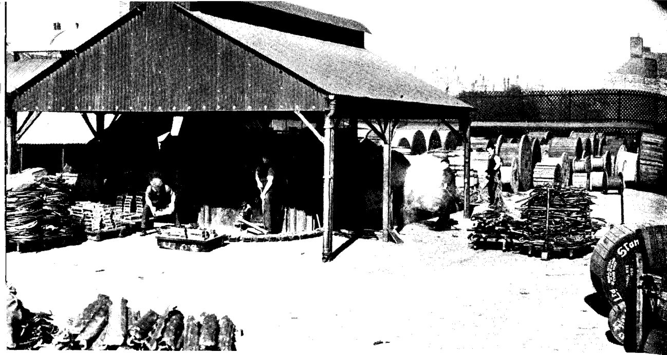
Kingsland Green Depot, London, melting plant
