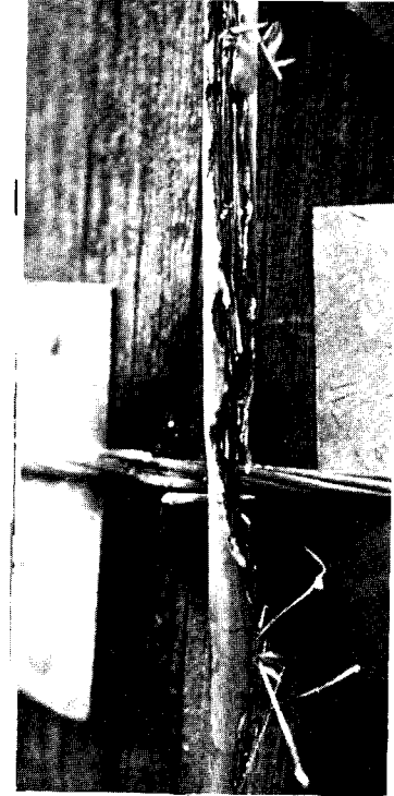
Fig. 4. Lead-in cable burst at exchange end. Test 1
