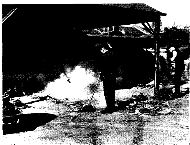
Drawing out red-hot copper wire from the melting pot
