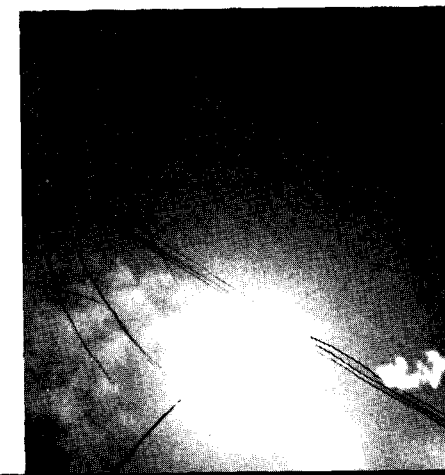
Fig. 2. Power conductor arcing and telephone wires breaking and arcing to each other. Test 3
