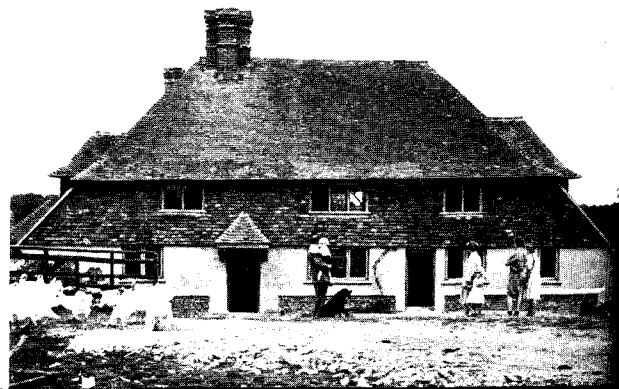
Wildage Farm under reconstruction
