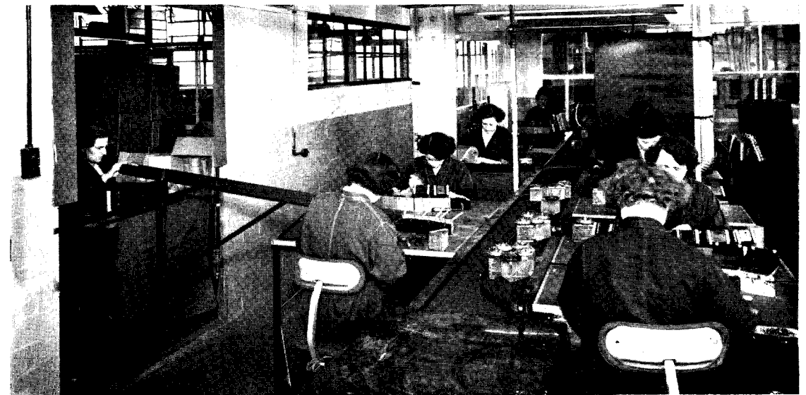
Flowline repair of telephone dials—dismantling line
