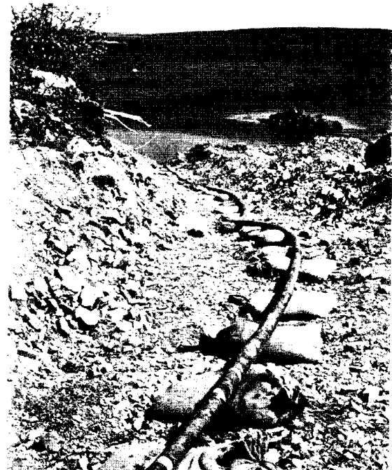
Cable coming ashore at Newfoundland
