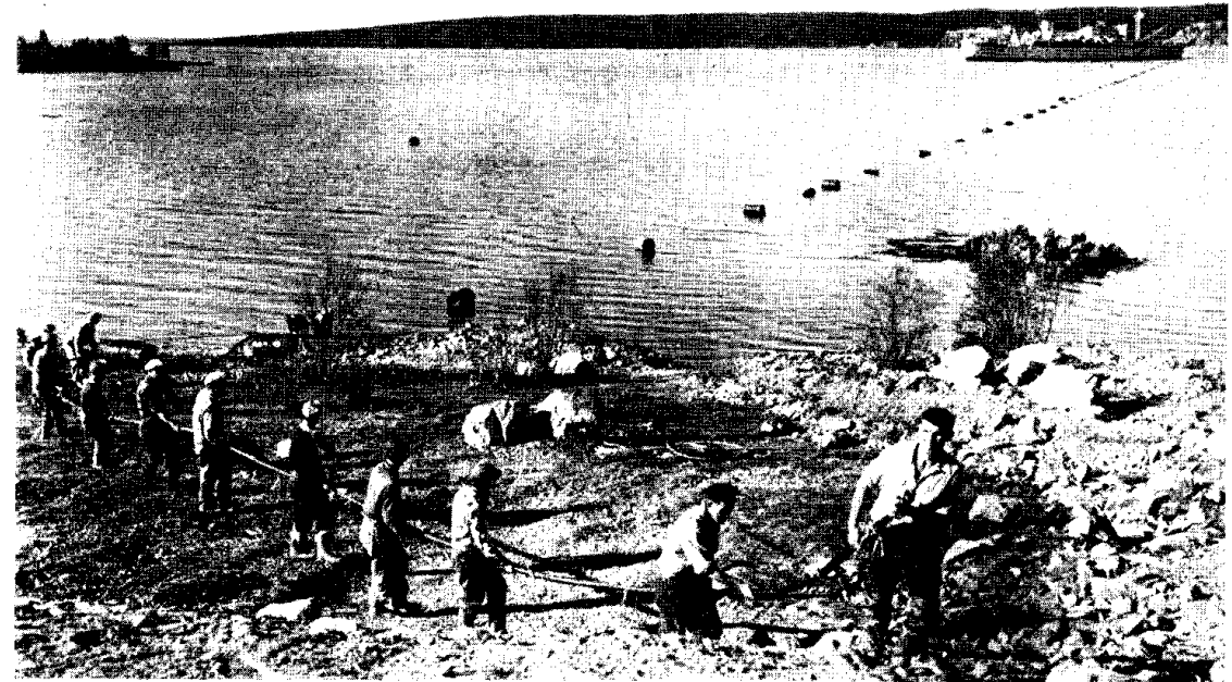
Hauling cable ashore from "Monarch" at Clarenville, Newfoundland
