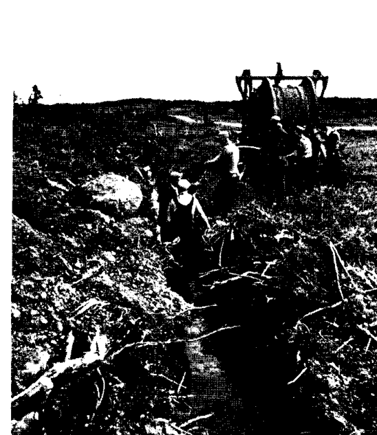
Cable laying in a flooded trench
