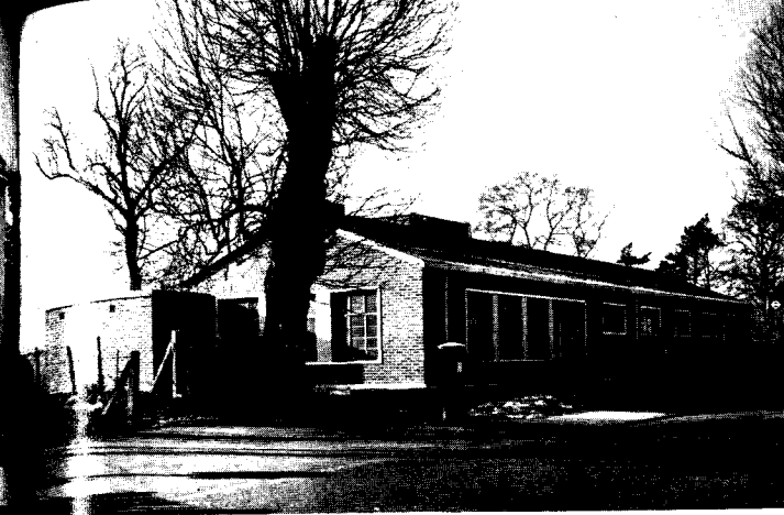
Above: Claygate Temporary Manual Exchange, Surrey. Standard concrete frame, asbestos roof and standard metal windows in precast stone surrounds
