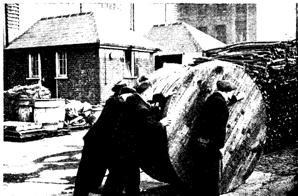
A comparison of methods for moving a drum of cable
