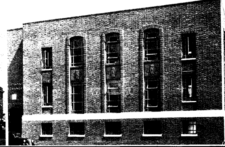
Below: Barnstaple Telephone Exchange, Devon. Brick building with a flat roof and a stone course at first floor-level
