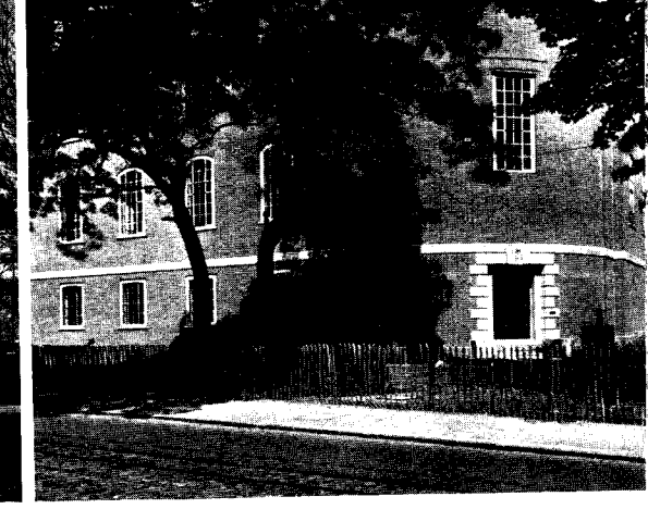
Above: Lee Green Telephone Exchange, London. Steel frame structure, solid brick walls, reinforced concrete floors and roof and metal windows in stone surrounds
