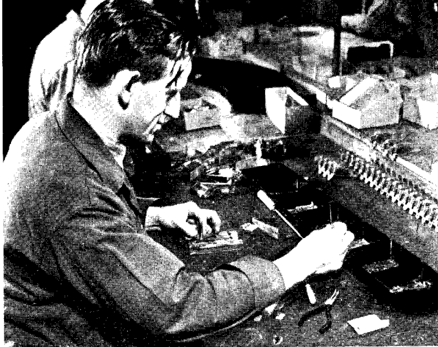
Assembling Relay Springs
