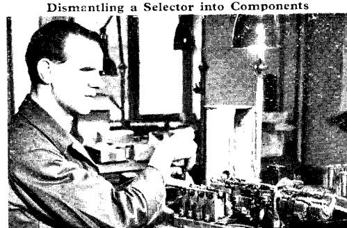
Dismantling a Selector into Components
