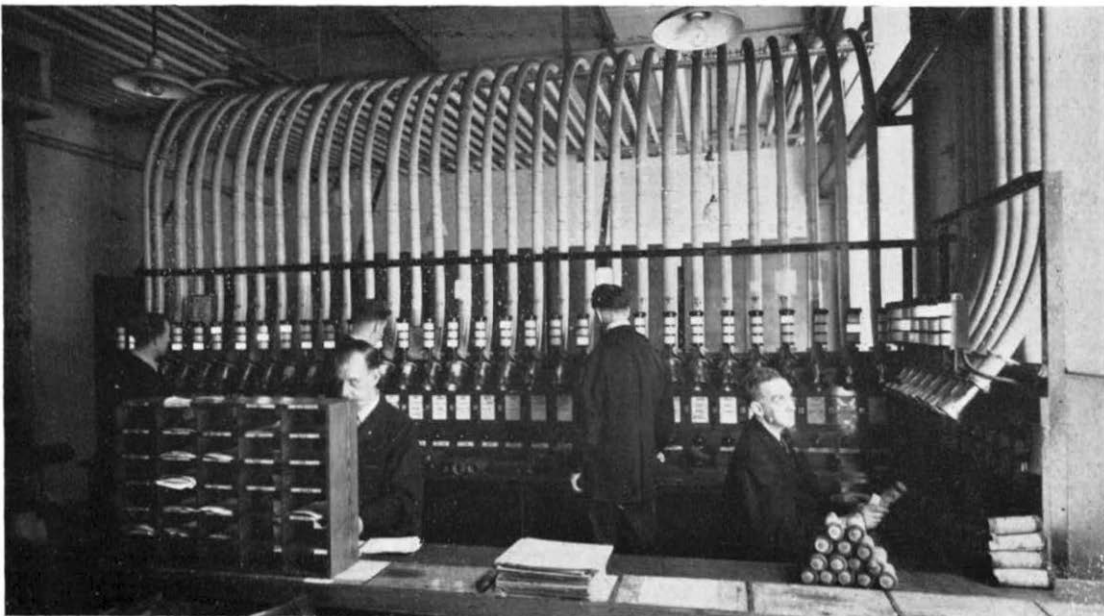
Outgoing tube terminals at Central Telegraph Office
