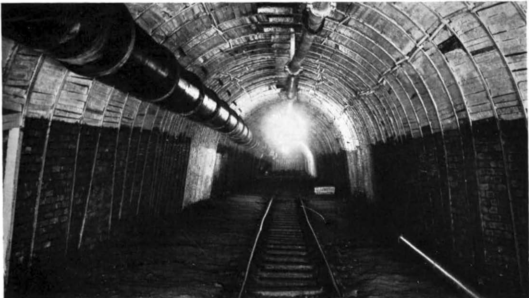
Below: Modern re-constructed underground roadway at Mardy Colliery, Rhondda Valley; this roadway, which must be close to the shaft bottom, is very uncommon as most roadways are dark and very restricted (Courtesy of South Western Division of N.C.B.)
