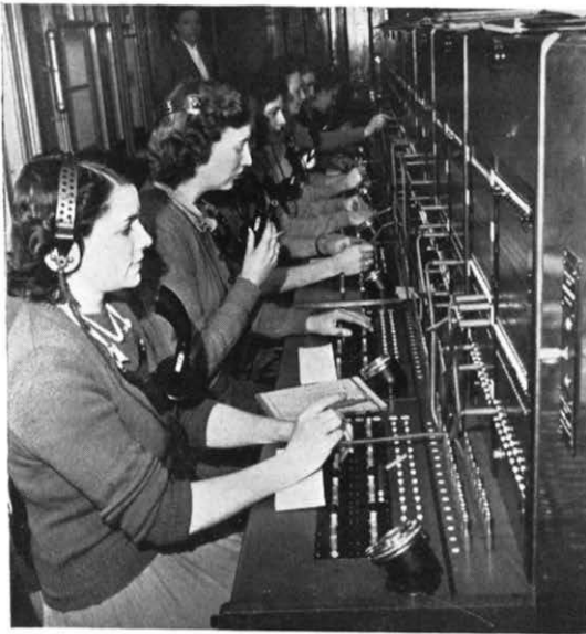
The P.B.X. switchboard at Divisional Headquarters
