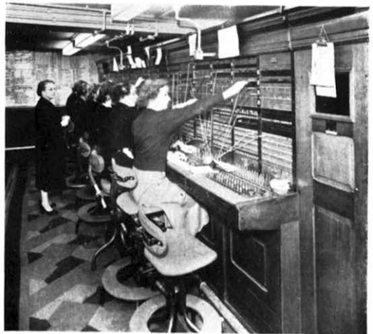
P.B.X. Switchboard at the Regent Palace Hotel
