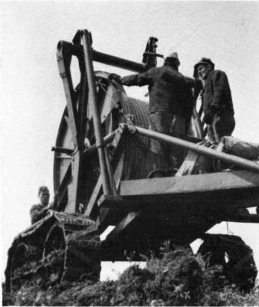
Ready for cable laying
