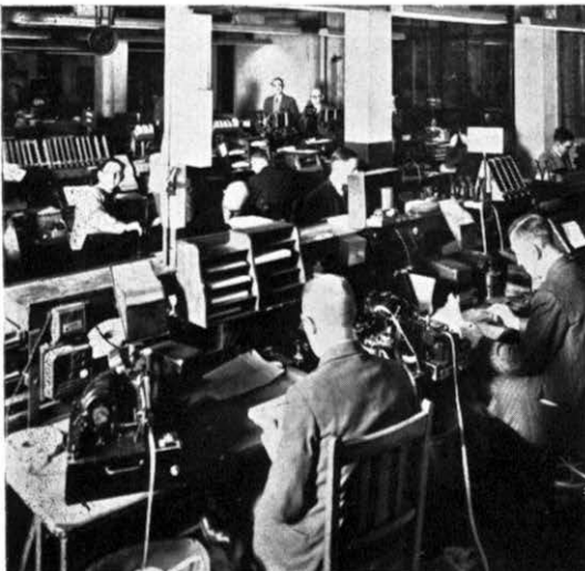
Section of the main operating gallery
