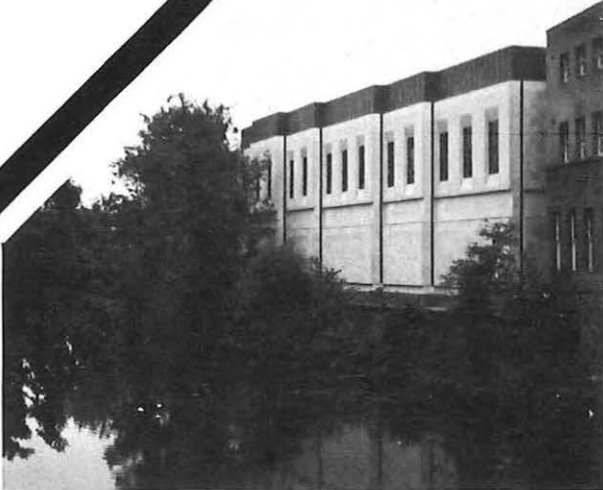
Refurbishment and new extension, B.P.O., Leamington Spa.
