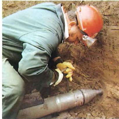
Final adjustments are made to the launching platform immediately before the machine begins work.
