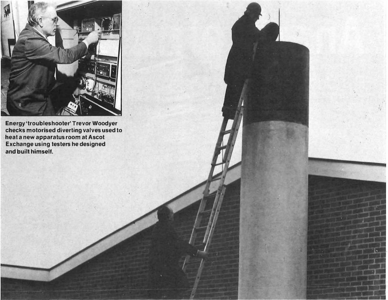
A rubber dustbin lid with a hole cut in it and placed over a boiler flue stack at Henley Exchange proved that the flue diameter was too large – thus leading to inefficient boiler firing.
