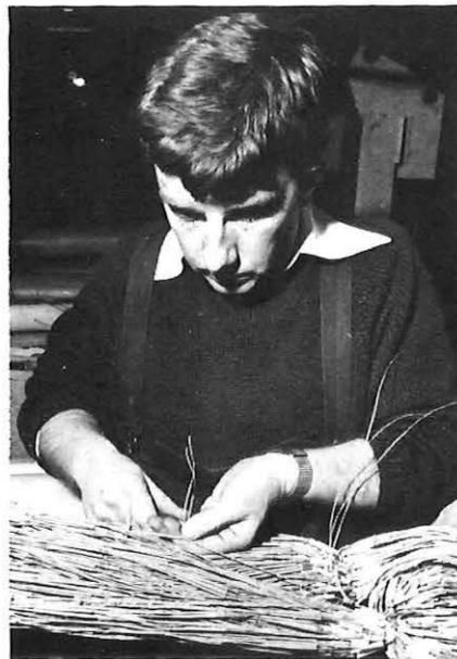
Nimble fingers are an asset in the repair of many telephone cable faults.
