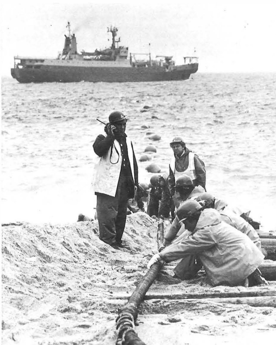
A new cable linking the UK with Spain was brought ashore by engineers from the Post Office cable ship Monarch on a lonely beach at Porthcurno, Cornwall in October. Able to carry 400 simultaneous telephone conversations, the new cable is by far the largest capacity undersea link to span the 423 nautical miles to Rodiles in north west Spain. It will also be used to relay messages to other European countries and will be interconnected with TAT7 – a new transatlantic cable due to come ashore on the same beach – early next year.
