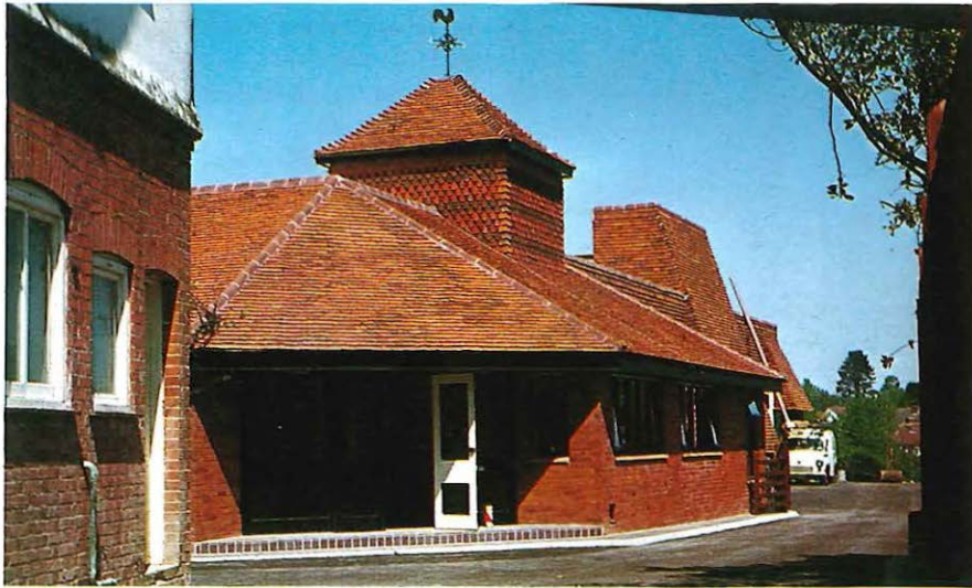
Cranbrook Exchange in Kent was skilfully designed to minimise the effect of its apparent mass in this attractive market town.
