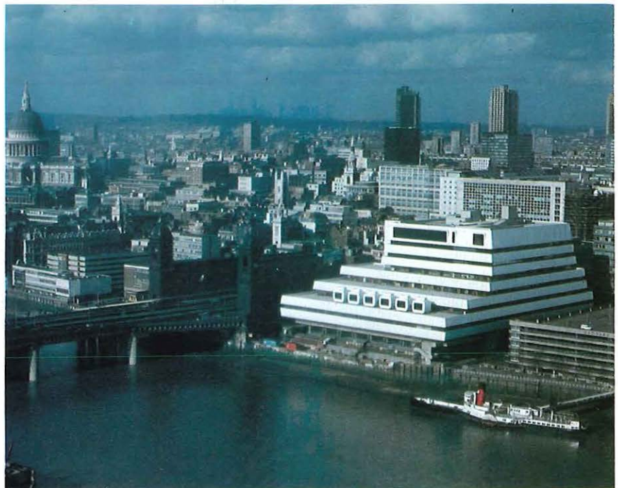
Mondial House – a distinguished architectural solution.
