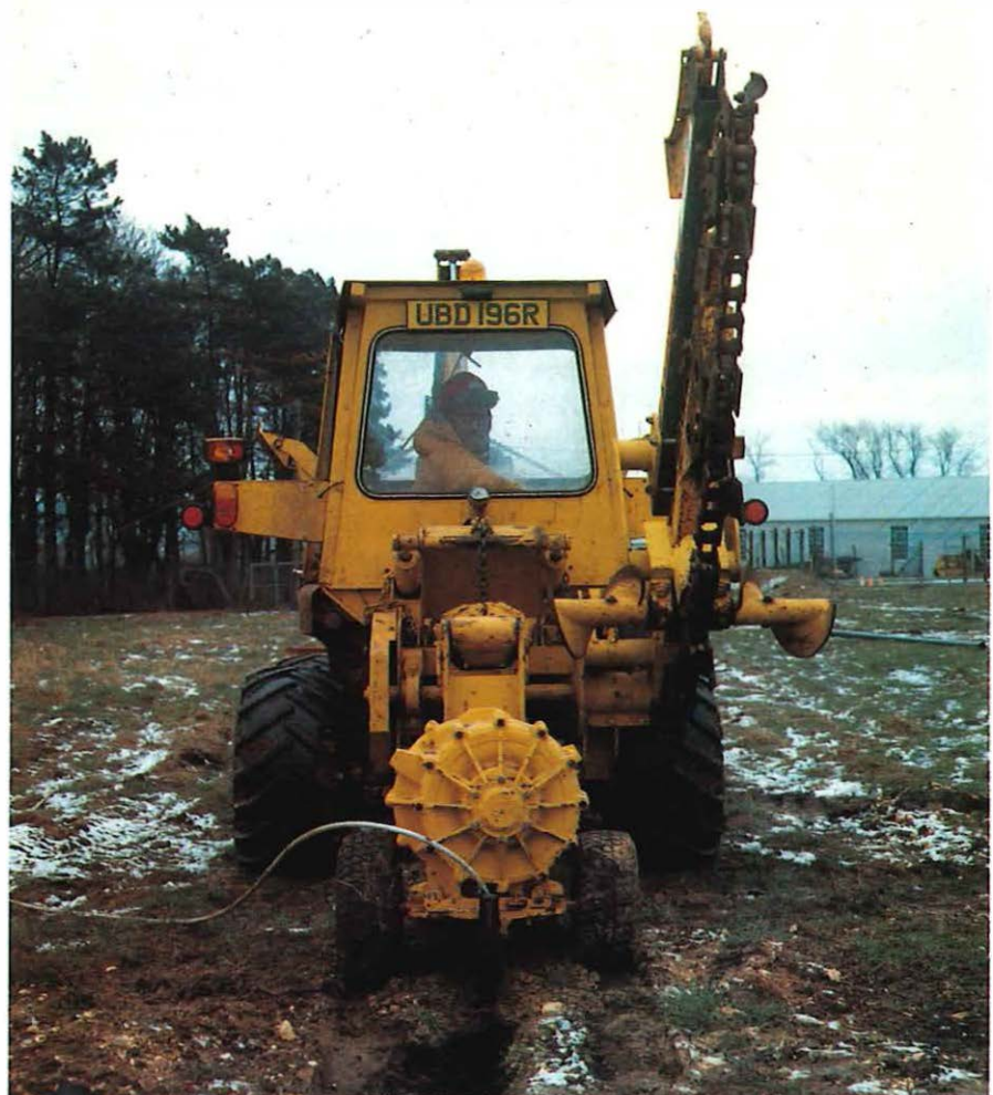
Cable is fed into the plough shoot of the Ditchwitch ...
