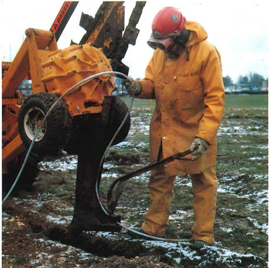
Cable is fed into the plough shoot of the Ditchwitch ...
