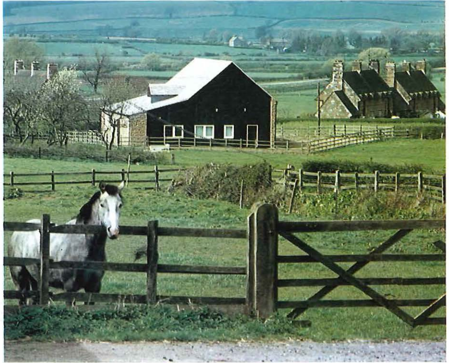
Rockingham, Northants, where a small modified telephone exchange complements the surrounding countryside Conservation Area.
