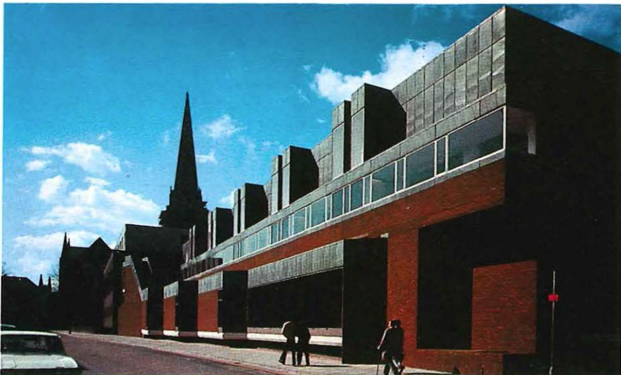
Chichester Telephone Exchange where an attempt to blend the sheer mass and scale of a large building into local surroundings has been undertaken.
