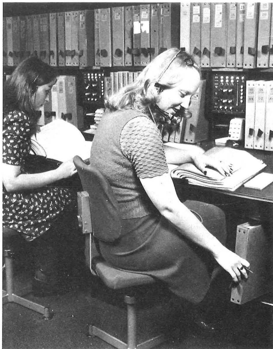
DQ operators working at Southampton-type sleeve control switchboards.
