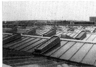
Smoke Ventilation Extraction equipment. Above: H.A.L. type. Right: 'Firelite' type
