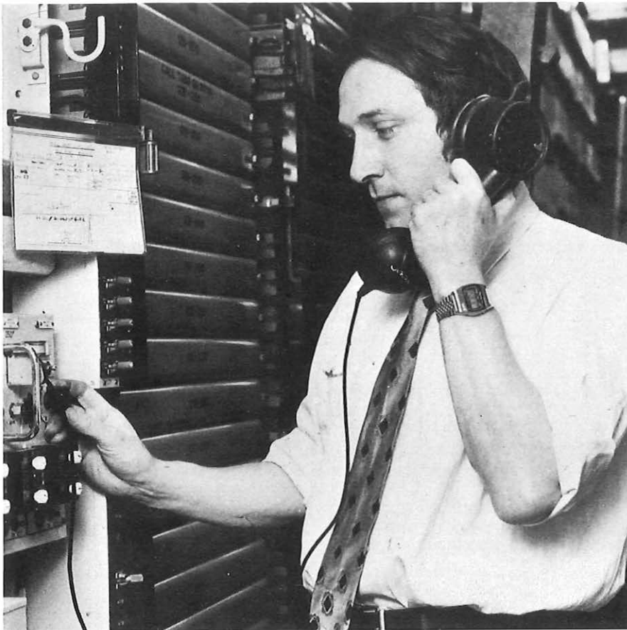
Technical officer Colin Dullighan checks the Radio City amplifiers at Liverpool Tandem Exchange.
