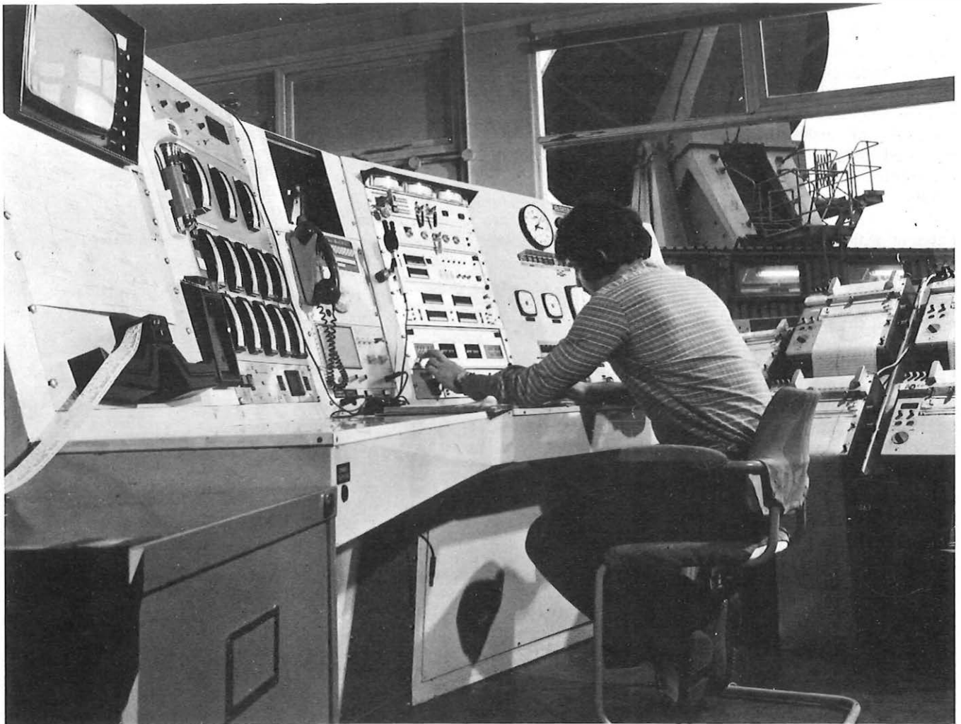
Roger Stuckey, Technical Officer on duty at the Cassegrain aerial control console manually controls the pointing angle of the aerial.
