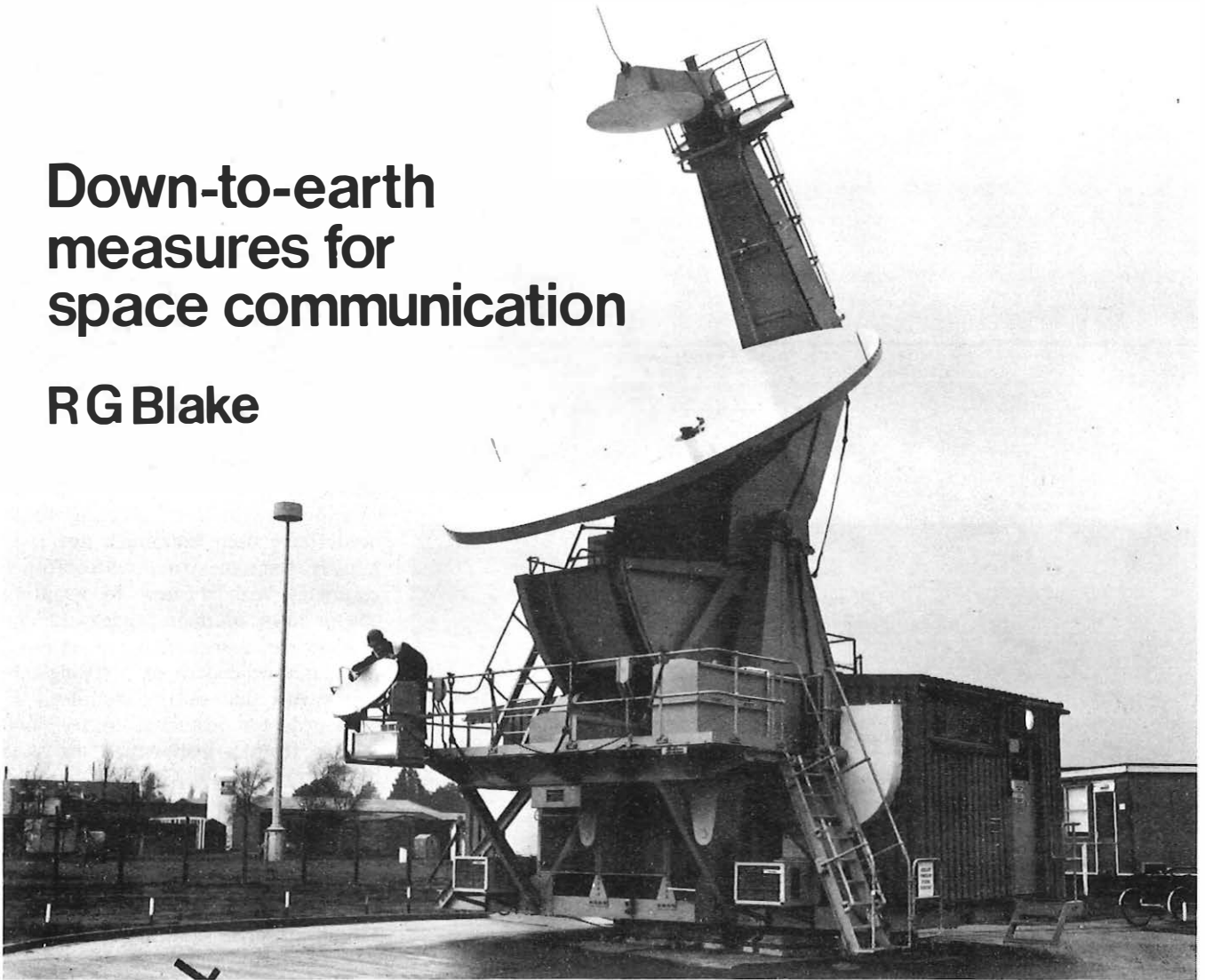
Nigel Gollin, AEE, makes an adjustment to the radar antenna mounted on the 6.1 m Cassegrain aerial at Martlesham
