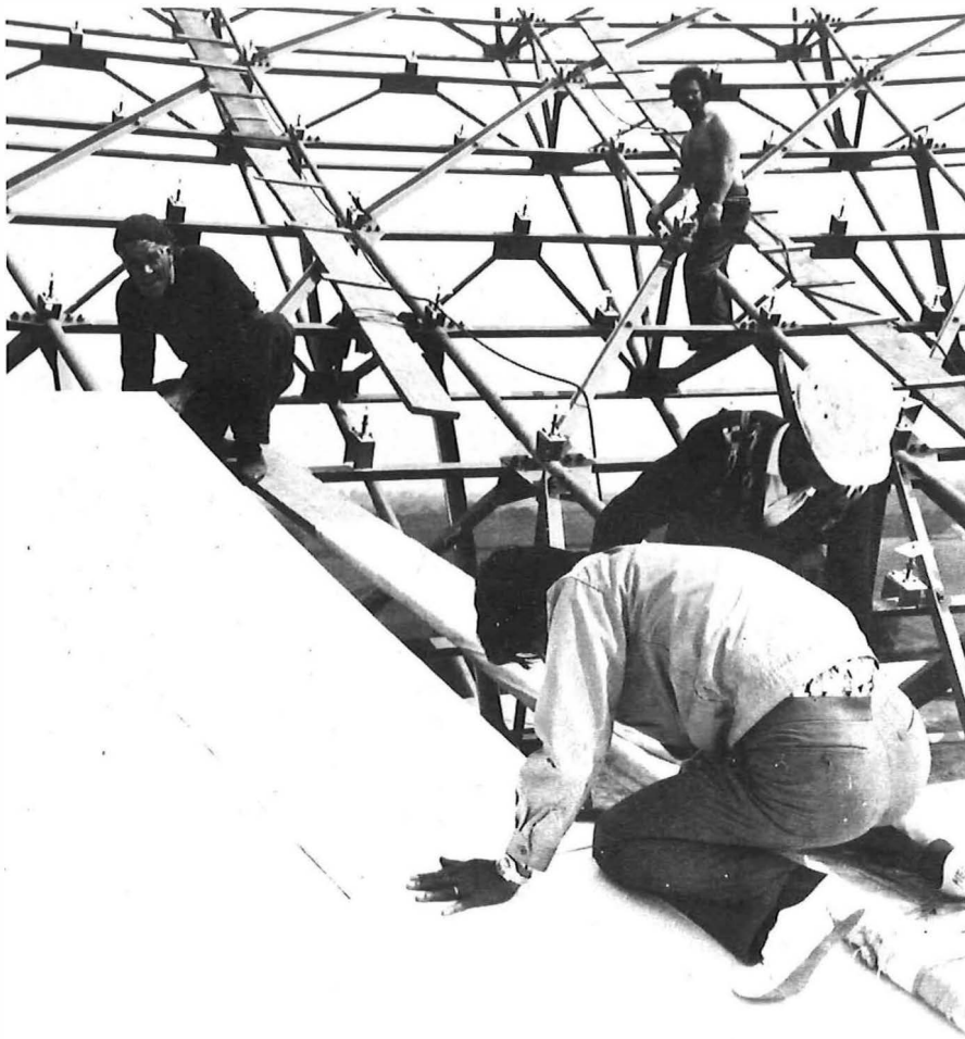
Contractor staff worked some 70 ft above the ground to fix aluminium panels to form the reflector surface of the aerial. The bolts projecting above the framework are used to adjust the surface within 1 mm of a true paraboloid.
