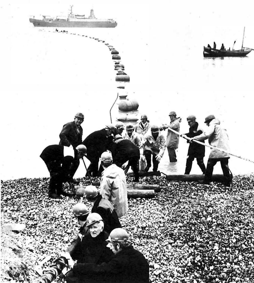
Mission complete: The UK-France cable is floated ashore at Eastbourne. In the background is Post Office cable ship Monarch.
