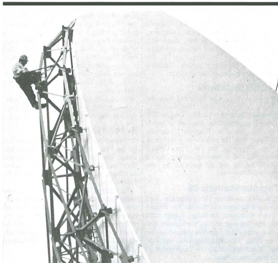
One of the team helping build the Post Office's new earth station at Madley, Herefordshire, works on the first aerial which could become operational later this year. It is hoped to carry an article on the new station in the Summer issue of the Journal.
