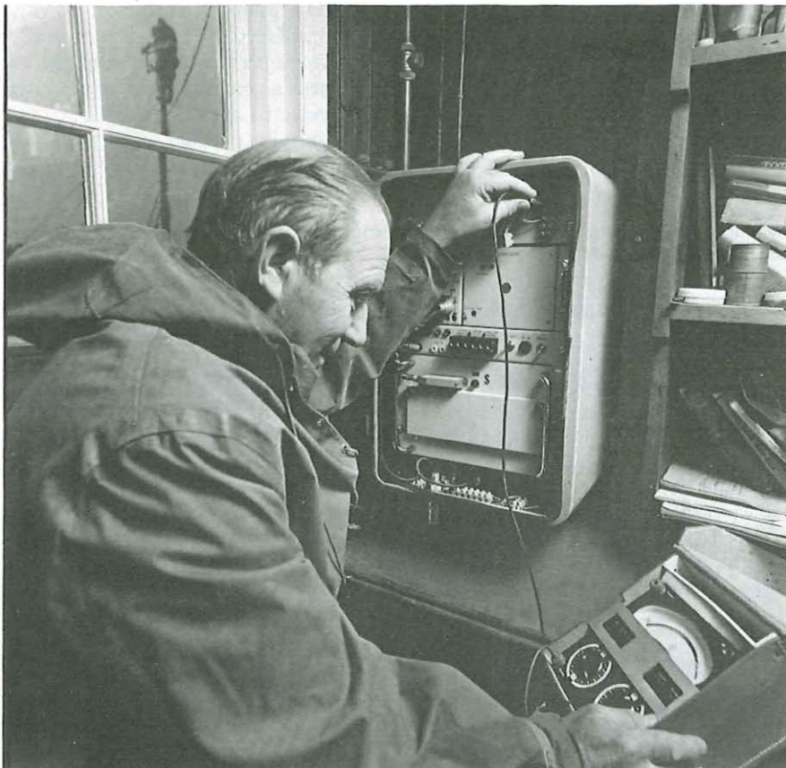
The output from a solar panel at Blakeney Point is checked on the radio-telephone transceiver by Assistant Executive Engineer Ken Durrant.
