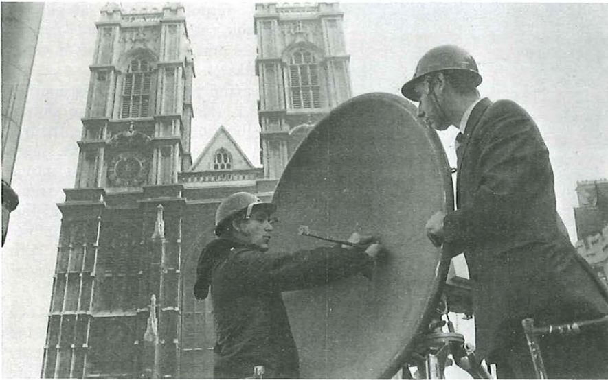
Assistant Executive Engineer Peter Cooke and Technician Joe Nicholls carry out transmission tests before live coverage of Princess Anne's wedding.
