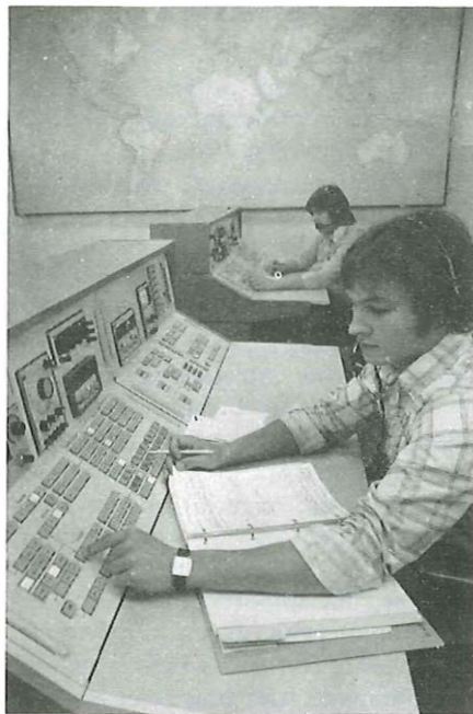
Technicians at the test desk of Stag Lane International Switching Centre in London check to ensure that directly-dialled calls are connected.
