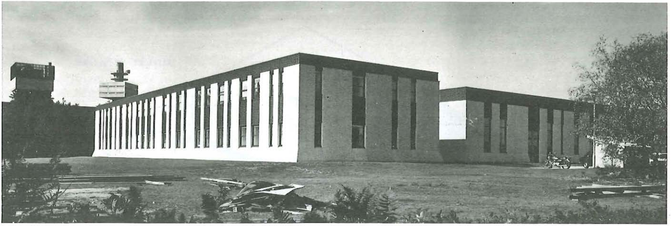
The switching system test facility building at the Post Office Research Centre.
