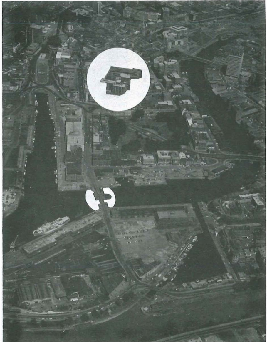
An aerial view of part of Bristol Harbour, showing the island area (centre, bottom) to which the new telephone cables had to be laid from the telephone exchange (top). A section was laid under water, alongside the swing bridge (centre).
