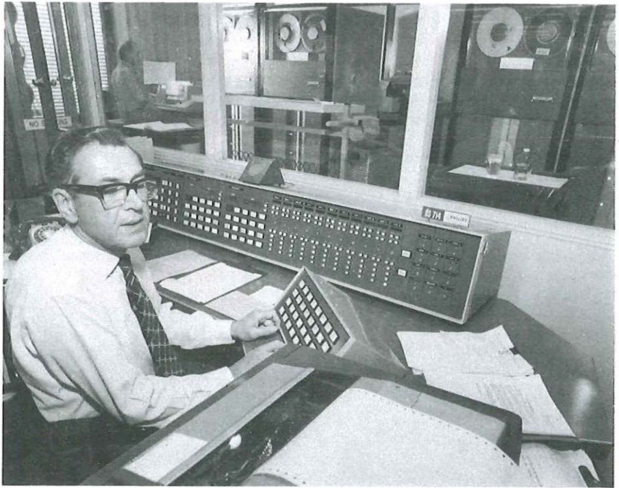
The message switching centre at the Shell Centre, which is connected to similar equipment in The Hague by way of telegraph channels superimposed upon the dedicated speech circuits for the desk-to-desk dialling facility.
