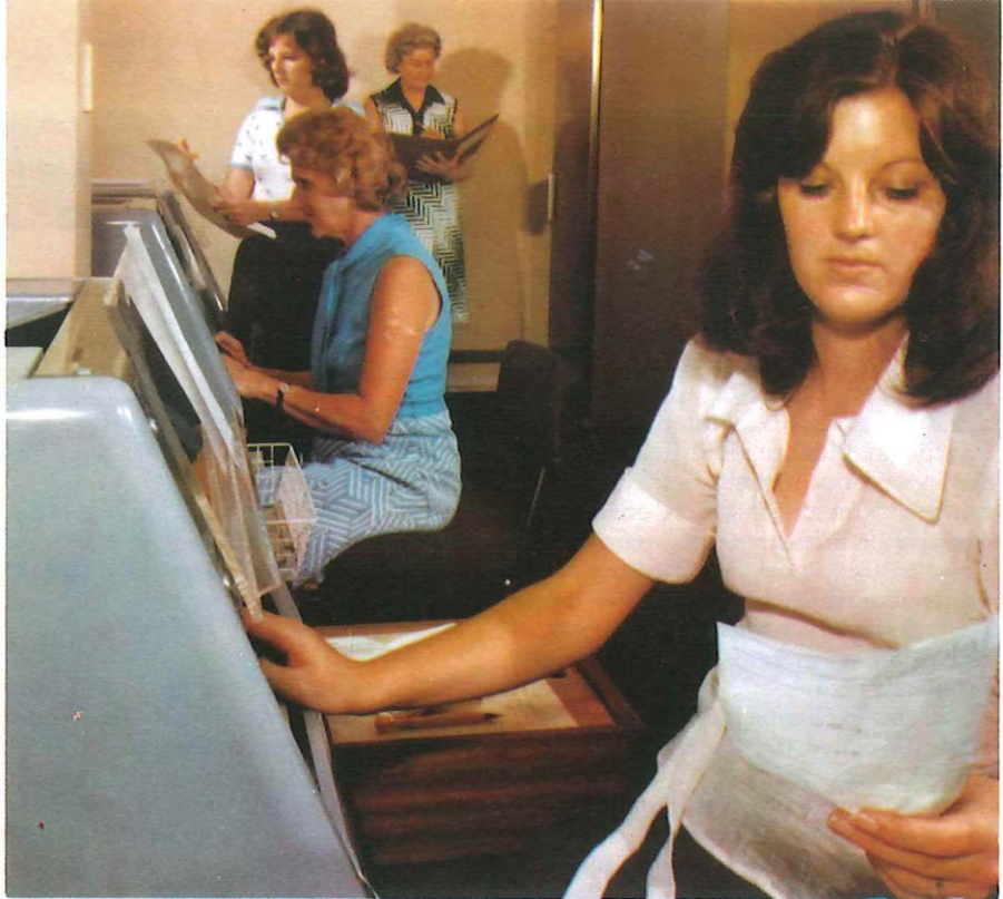
A bank of teleprinters at a customer's premises showing how the new PATBX equipment cabinet, in the background, blends easily into the office environment.
