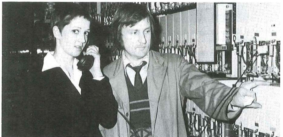
Michelle Salle receives some practical instruction from Technical Officer Colin Sharp at a City Telephone Area exchange in London.
